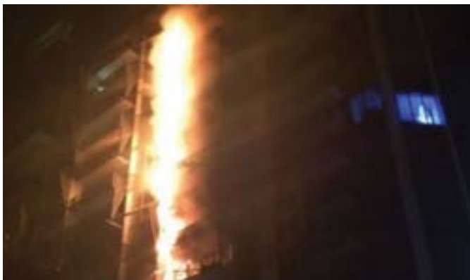
The 2014 fire at the Lacrosse tower in Melbourne's Docklands spread across the facade in a matter of minutes. Gregory Badrock/Metropolitan Fire Brigade Photo.
