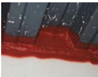
Firestop spray system at head of wall. Zussman/Pepper Photo
