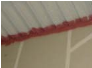
Spray fireproofing (SFRM) on deck. Fire Stop Technologies Photo
